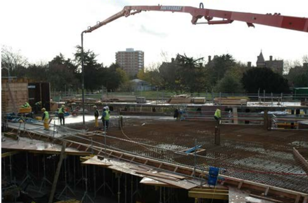
Pouring concrete for the first floor
