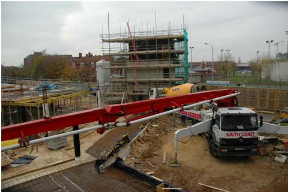
Long range concrete pouring
