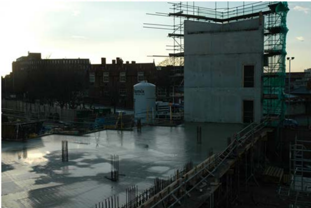
First floor concrete poured and still wet
