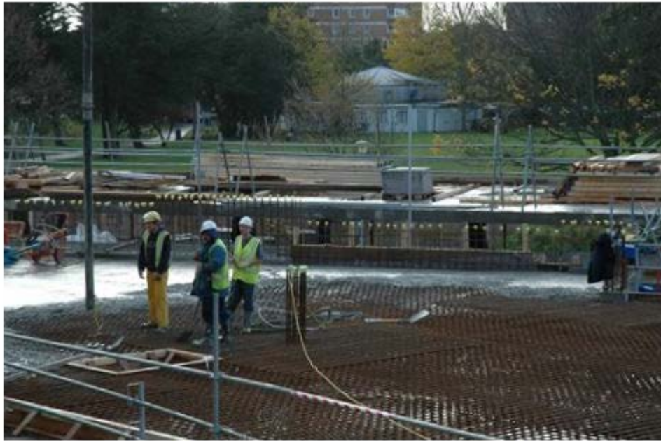
First floor concrete poured and still wet
